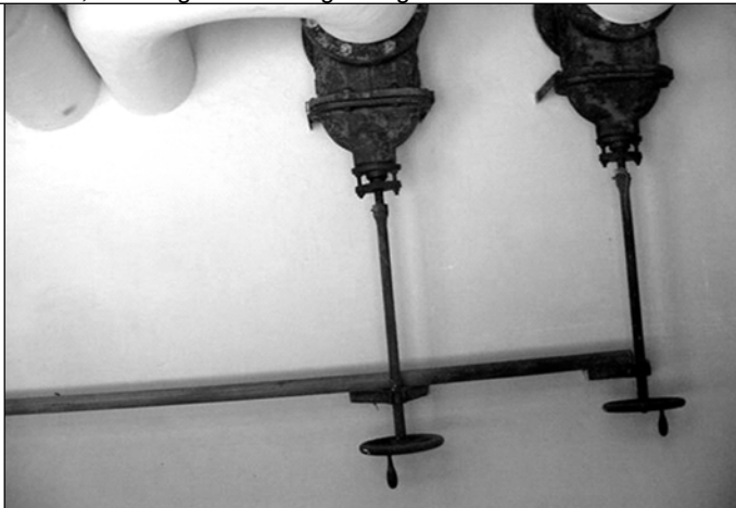
Fig. 51: Heavy insulated hot water (or steam?) pipes in the room behind the alleged gas chamber of Dachau camp, leading into the space above the current room. 1
