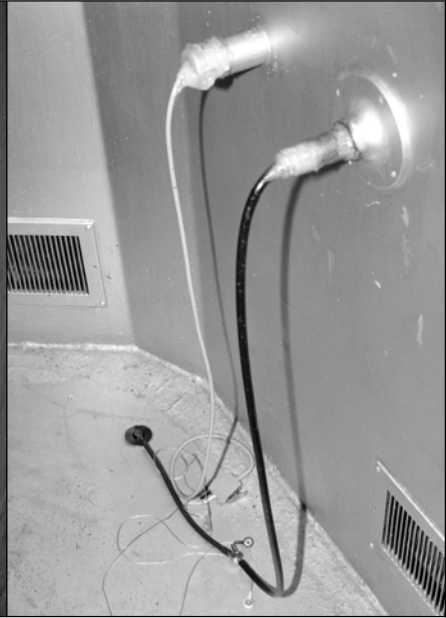
Fig. 97: Inside gas chamber where stethoscope and other body monitoring line enter. They are covered in vaseline to indicate leaks. Fresh air vents on the walls close to the floor.
