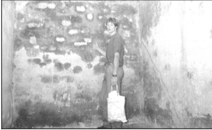
Fig. 38: Blue staining of the Interior northwest room in the Zyklon B disinfestation wing of BW 5a in the Birkenau camp. (© Karl Philipp 201 )
