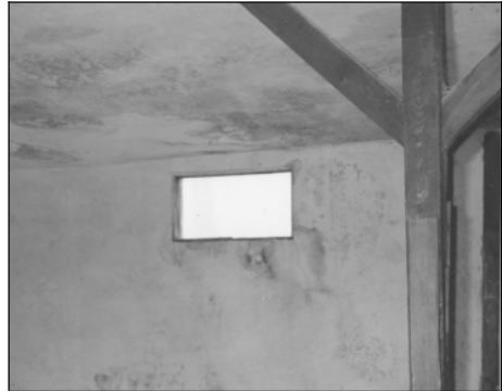
Fig. 30: Window in chamber IV of building no. 41 (alleged homicidal gas chamber, but actual delousing chamber), Majdanek camp. © C. Mattogno
