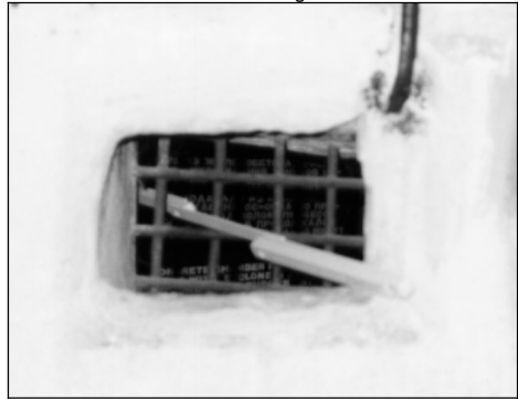
Fig. 33: Opening with grate in the wall of room I in the disinfestation wing of building 41, Majdanek (see Fig. 31) © C. Mattogno
