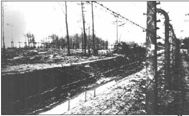
Fig. 5: Drainage ditch running north of Crematorium V 25
