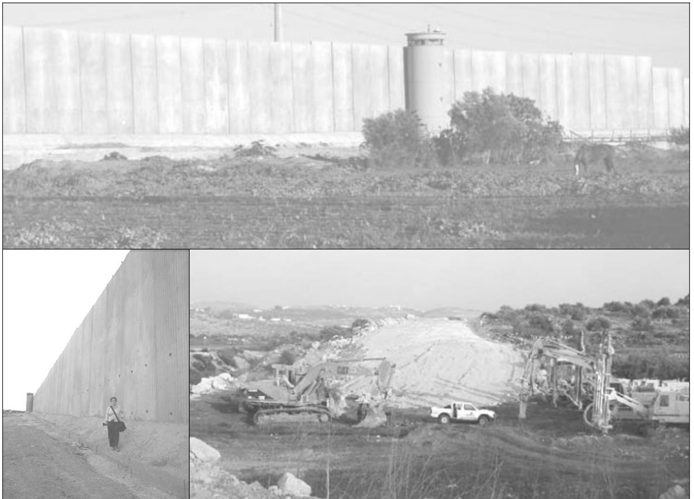
The Gaza Wall, Israel's Anti-Arab Defence Wall, under construction...
